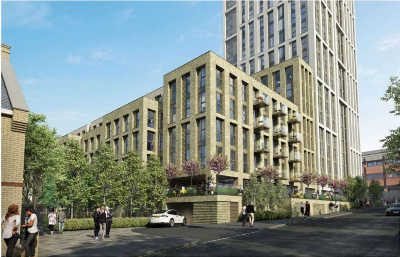
St John's Road - West
